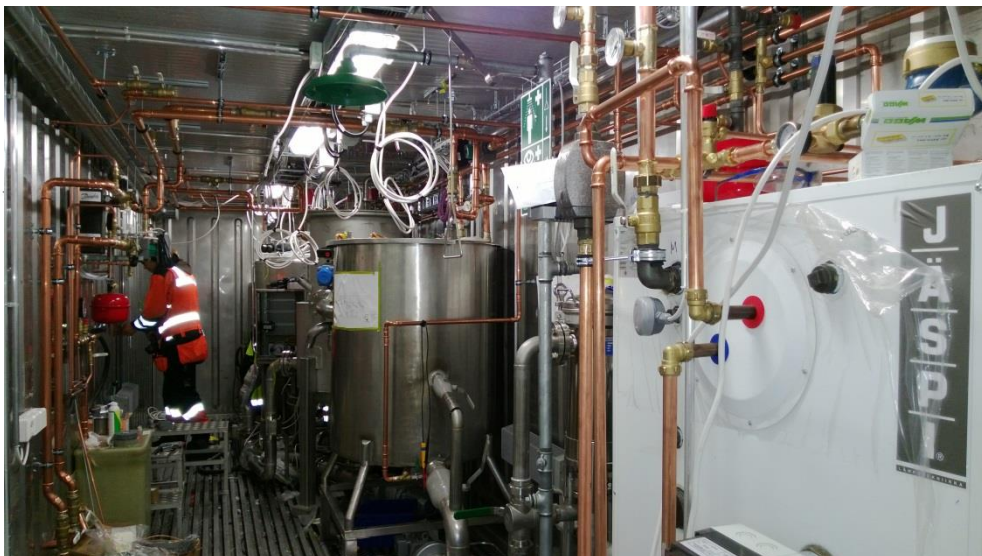
Process room of Pilot A during installations.
