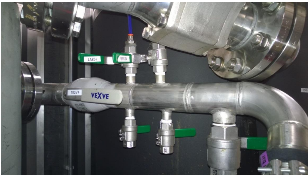
Picture 21 Sampling point in the bioreactor's circulating tube.
