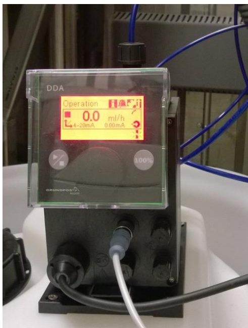
Picture 9 pH adjustment pump.
