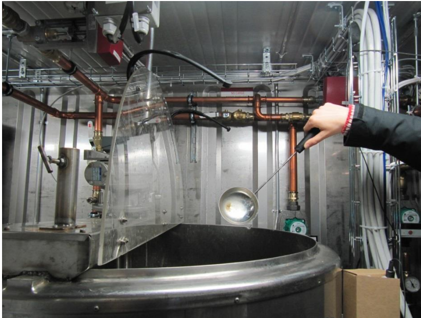
Picture 20 Sampling point in the hydrolyzer.
