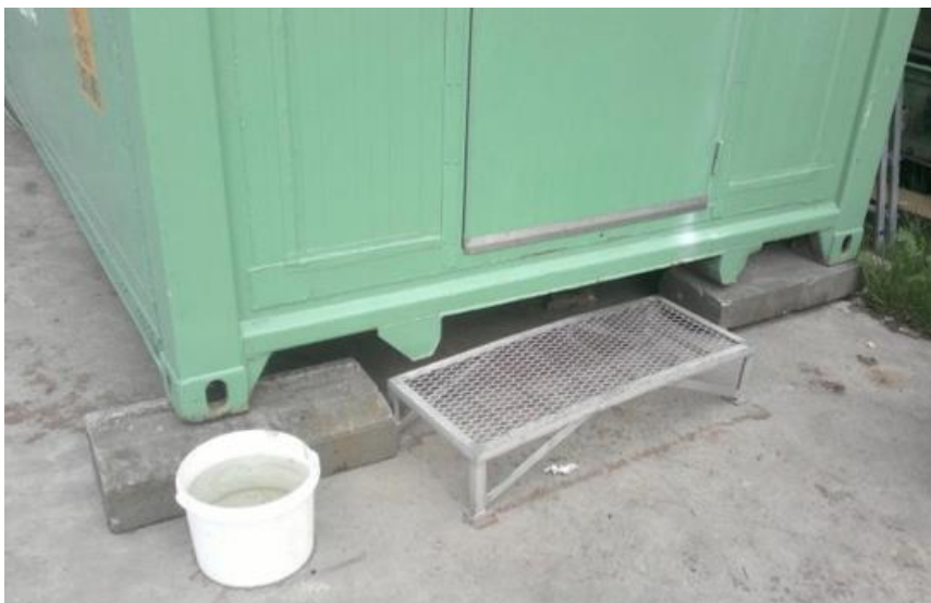
Figure 3: Levelling of the container with stone slabs.
