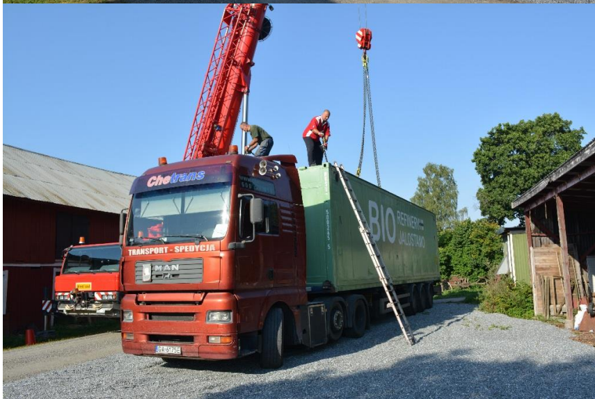
Figure 2: Unloading of the container in Sweden at Hagby gård Enköping.
