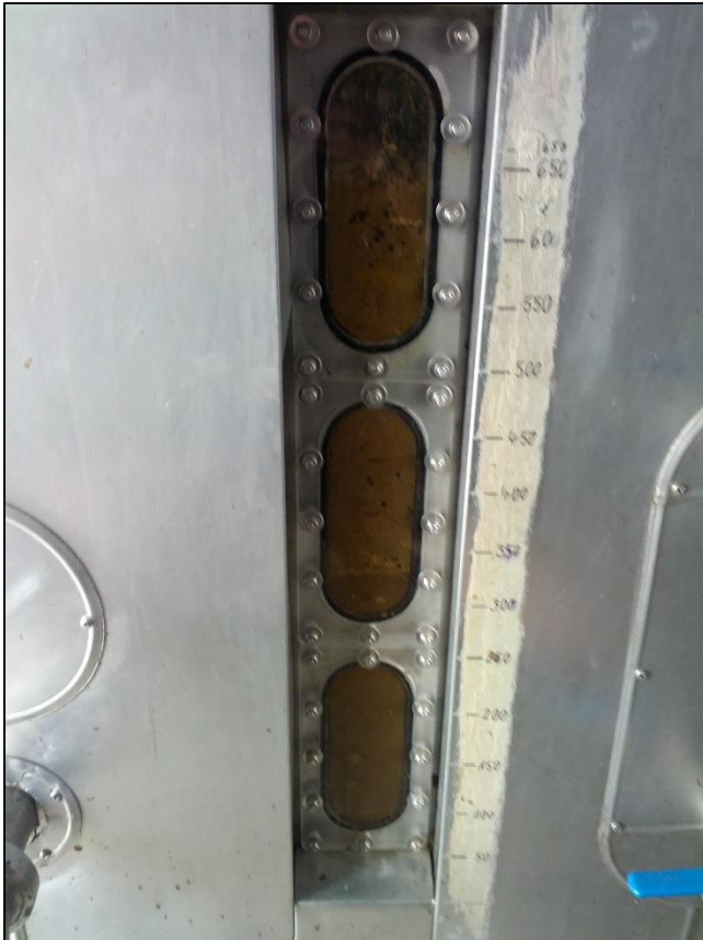
Figure 7: Openings in the fermenter wall to observe the fermenter content.
