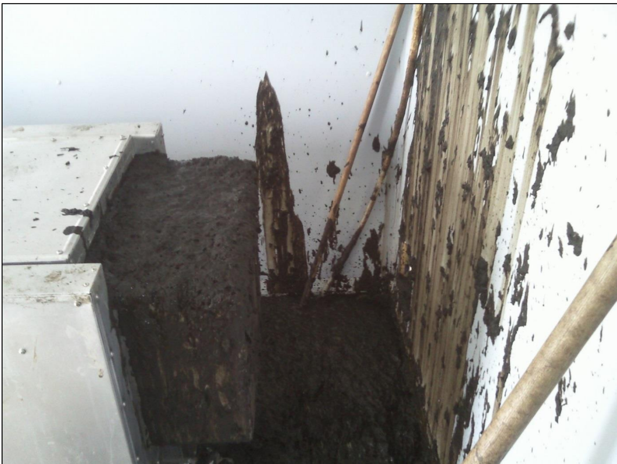
Figure 48: Spilt fermenter content after a longer electrical shutdown of the fermenter.
