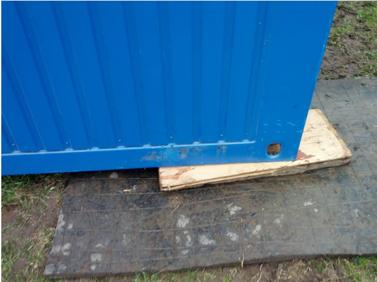
Figure 5: Levelling of the container with wooden boards.
