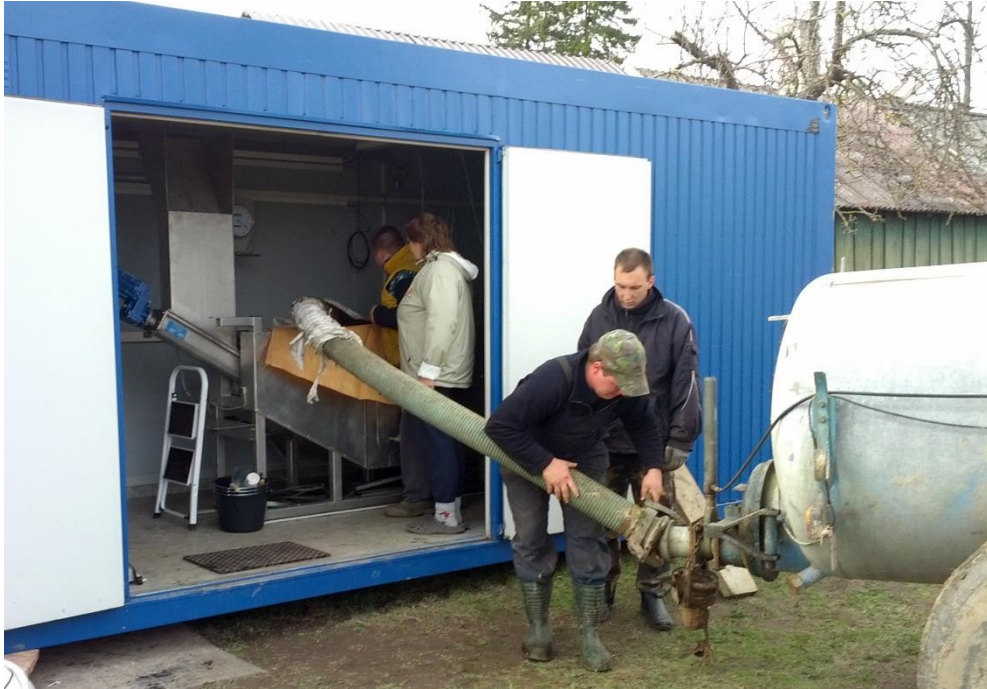
Figure 19: Initial filling of the fermenter with the help of a manure pump.
