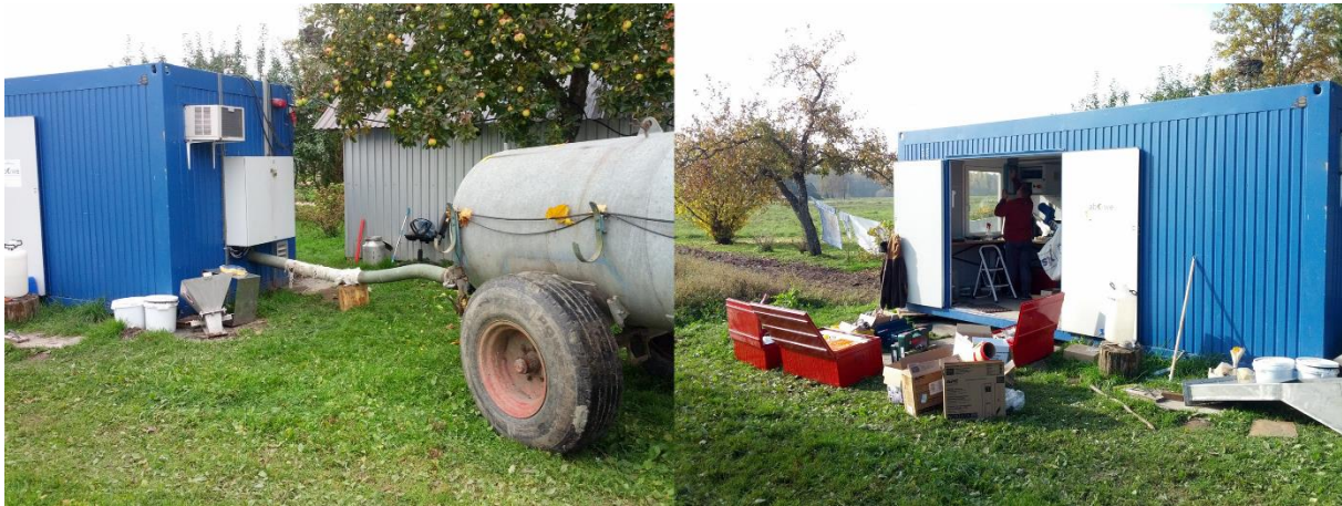
Figure 28: Removing of the fermenter content using a manure pump (left). Inventory control and sanitation of the pilot plant (right).
