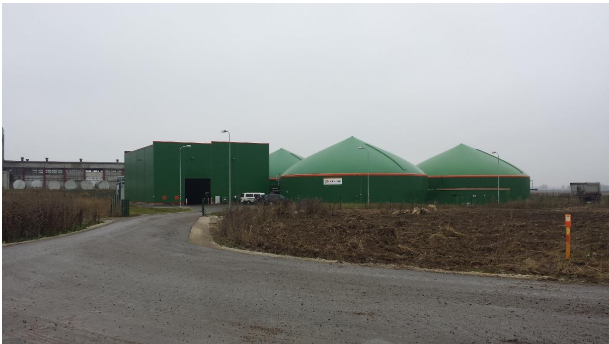
Figure 38: Estonian biogas plant, Vinni, Estonia, October 2013
