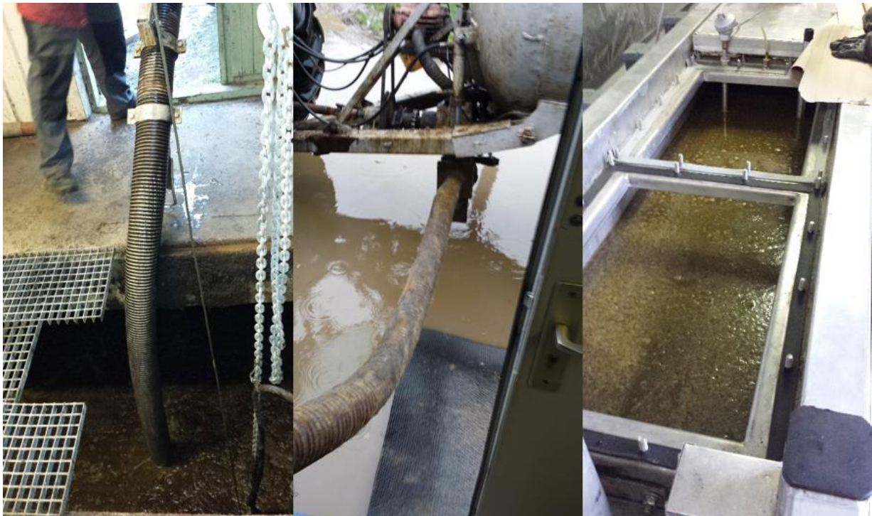
Figure 8: Initial filling of the fermenter. Pumping from the slurry pit, Filling with manure pump, Filled fermenter (left to right).
