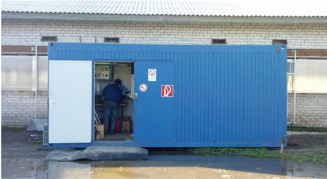
Figure 6: Levelling of the container with rubber mats.
