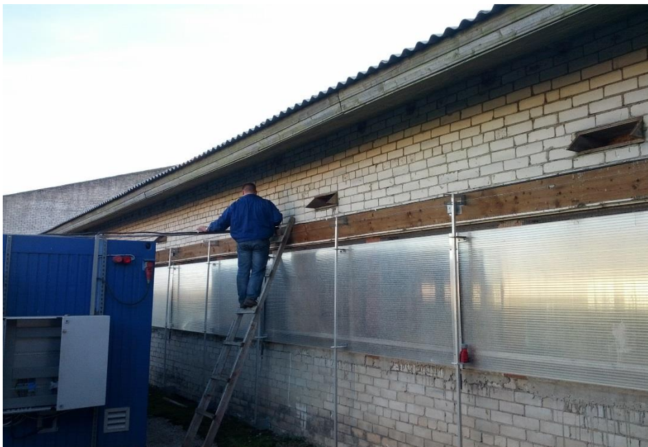
Figure 7: Connecting the pilot plant to the local electricity grid.
