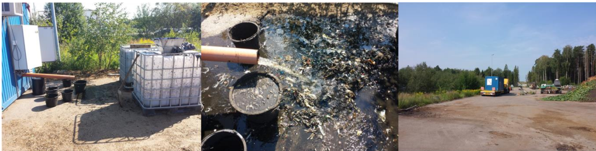
Figure 23: Impressions of the plant shutdown in Sweden. (left) Manual emptying of the fermenter with buckets. (center) Flushing with water to remove sediments. (right) Pilot plant on its way back to Germany.
