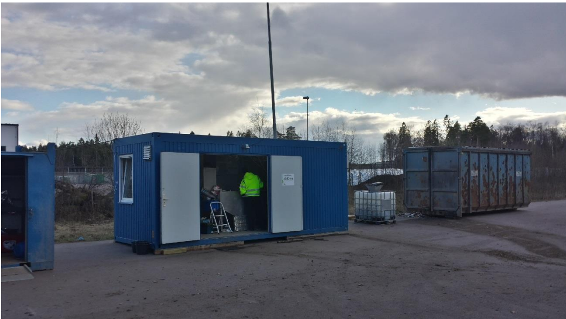
Figure 4: Levelling of the container with square timber.
